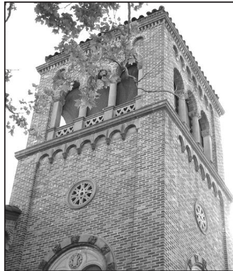
As Building B comes down, the bell tower will stay up.
