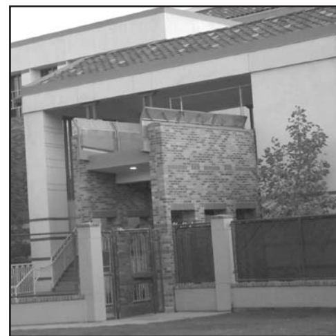
NOT LIKE THIS: Beverly Vista’s “Bridge to Nowhere”
