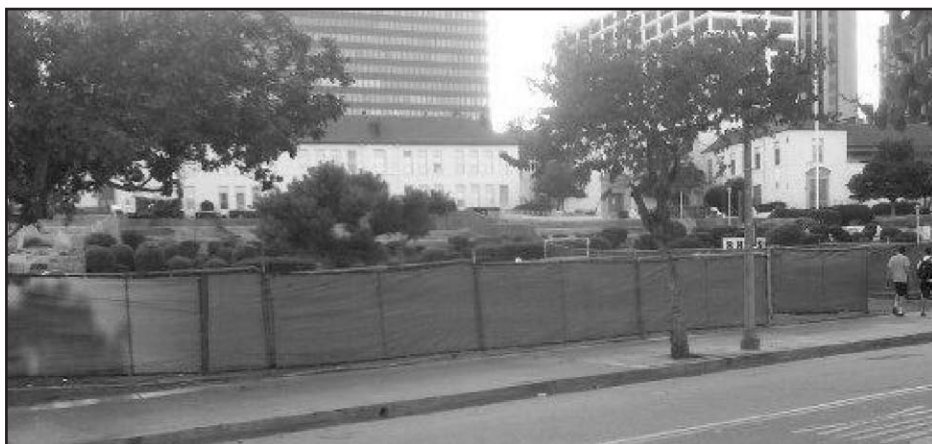
Temporary fences line Beverly High's campus for seismic testing and trenching
