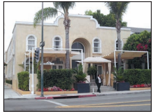
Existing Crescent Hotel
