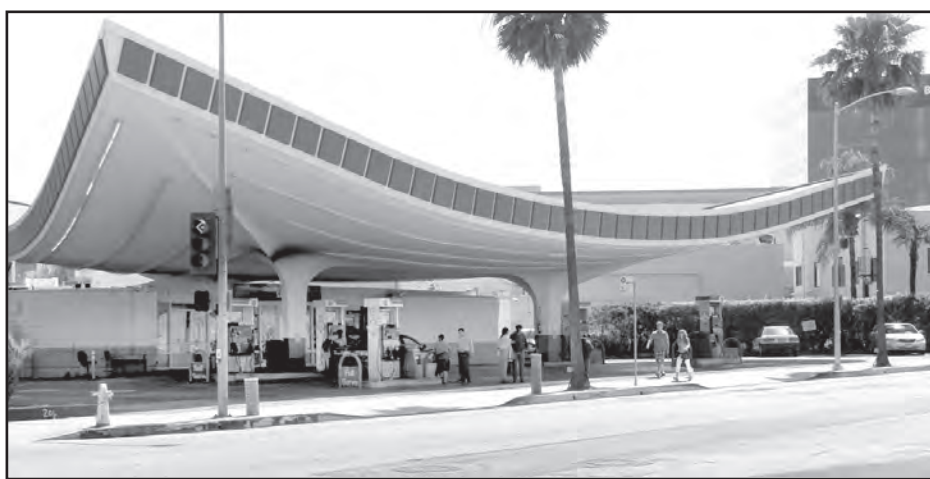
Union 76 gas station
