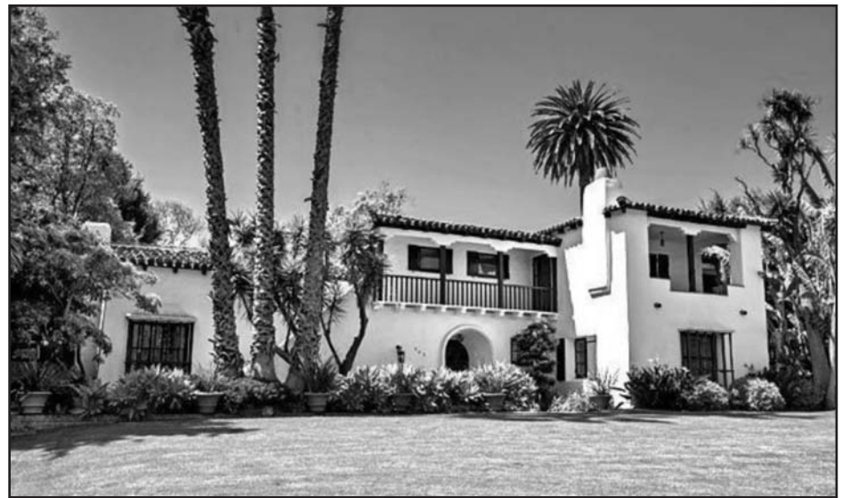
The property owners of 805 N. Linden Drive have applied for a demolition permit
