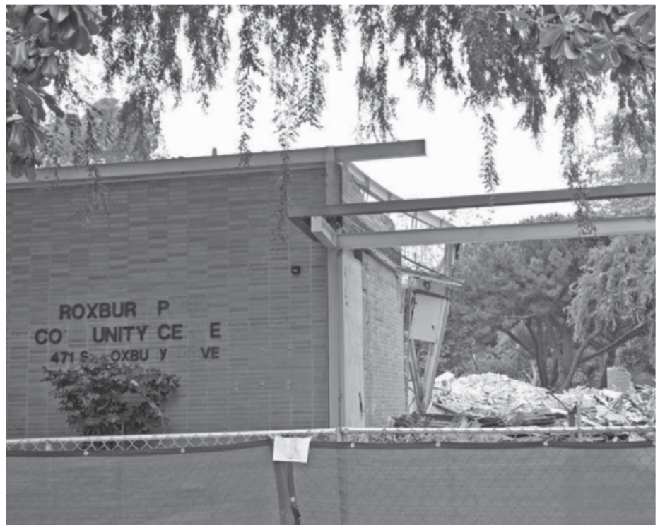
Roxbury Park Community Center during demolition
