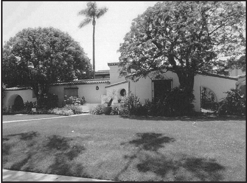
707 Walden Drive residence
