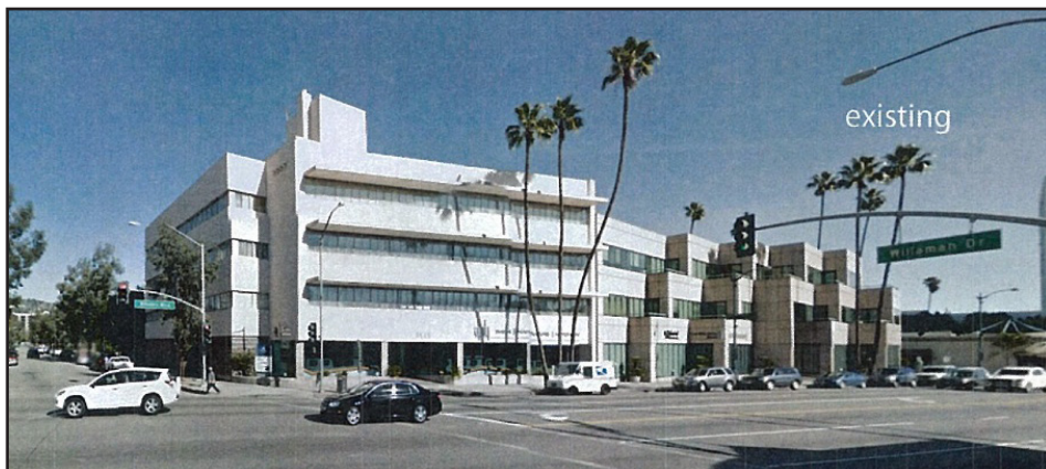
Current 8665 Wilshire building
