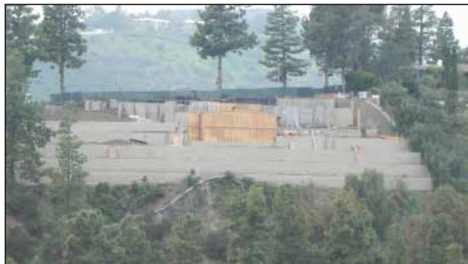
Retaining wall in the Hillside area
