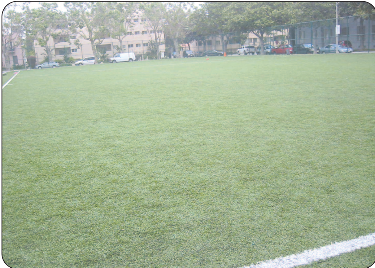
Recently-installed synthetic turf at Beverly Vista.
