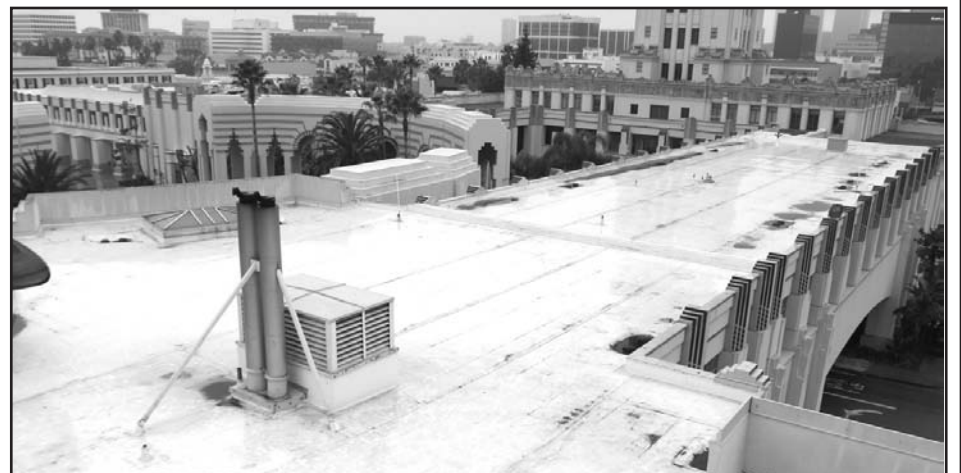
Solar panels will be installed on top of the Civic Center to generate clean energy.
