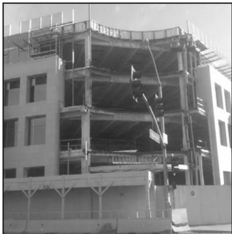
8767 Wilshire Blvd., during construction
