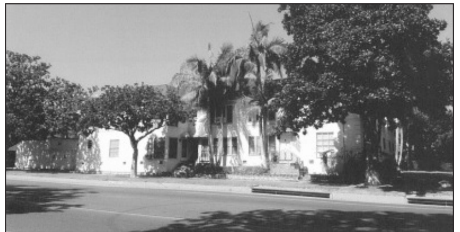
Existing residential building at 425 North Palm Drive
