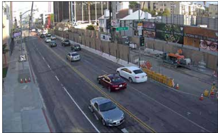
Piling on Wilshire between Gale and La Cienega
