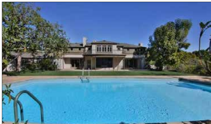
Existing property at 901 Whittier Drive
