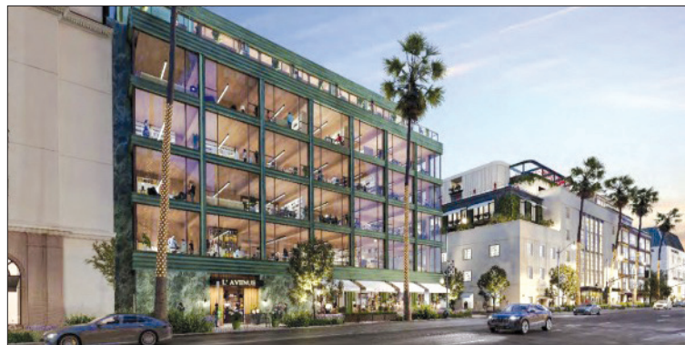
Example of Project from Wilshire Boulevard toward South Peck Drive
